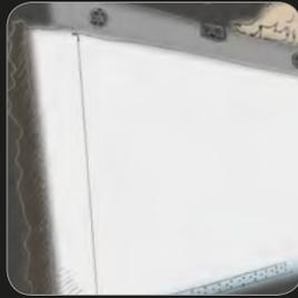
board covered with adhesive on the angle section and push (floating). Use a spirit level to check that it is level.
